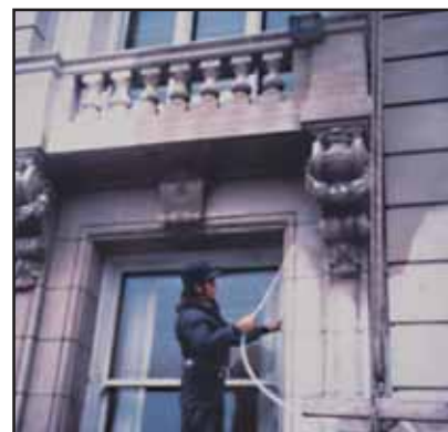
Figure 6. Spray application of silanes on large structures.
