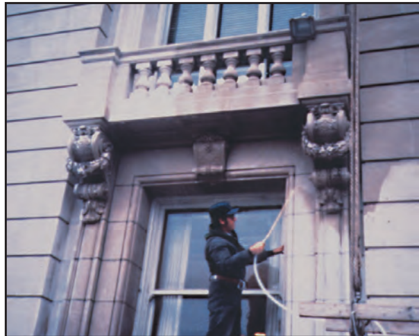
Figure 6: Spray application of silanes on large structures.
