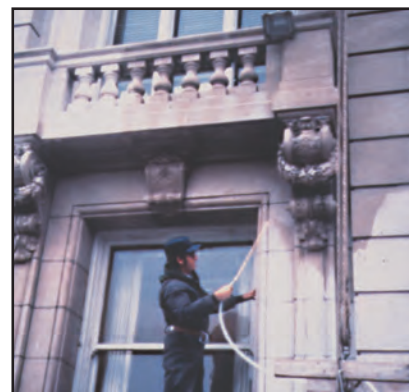
Figure 6. Spray application of silanes on large structures.
