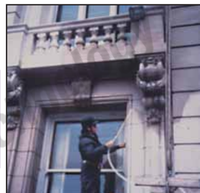
Figure 6. Spray application of silanes on large structures.
