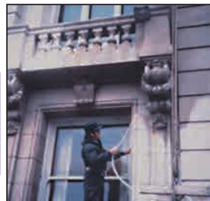
Figure 6. Spray application of silanes on large structures.
